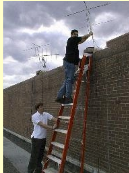
Gabe Fossati and Atul Pkharel mounting an antenna on the roof.
