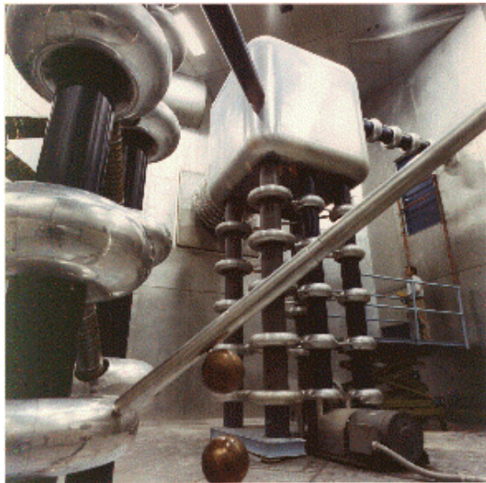
“Preac” - Static Cockroft-Walton generator accelerates H- ions from 0 to 750 KeV.
